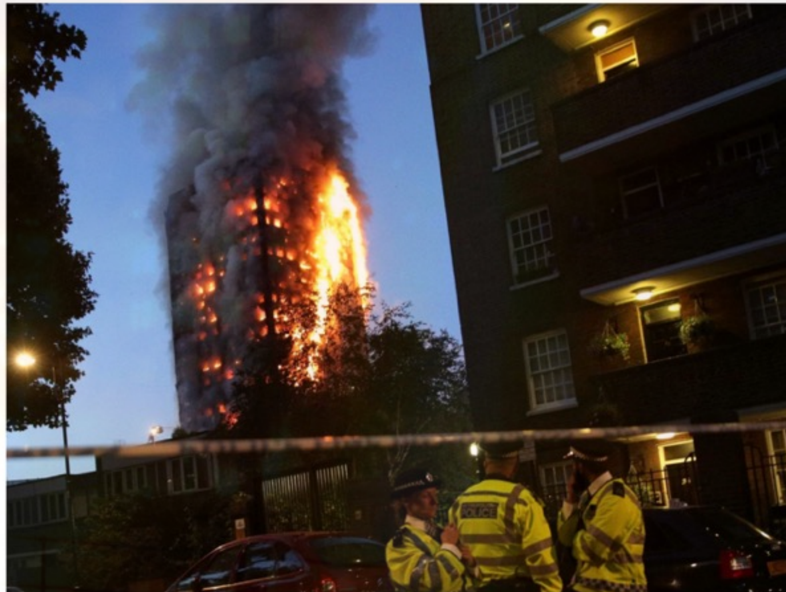
Fire engulfing Grenfell Tower in London on June 14.
