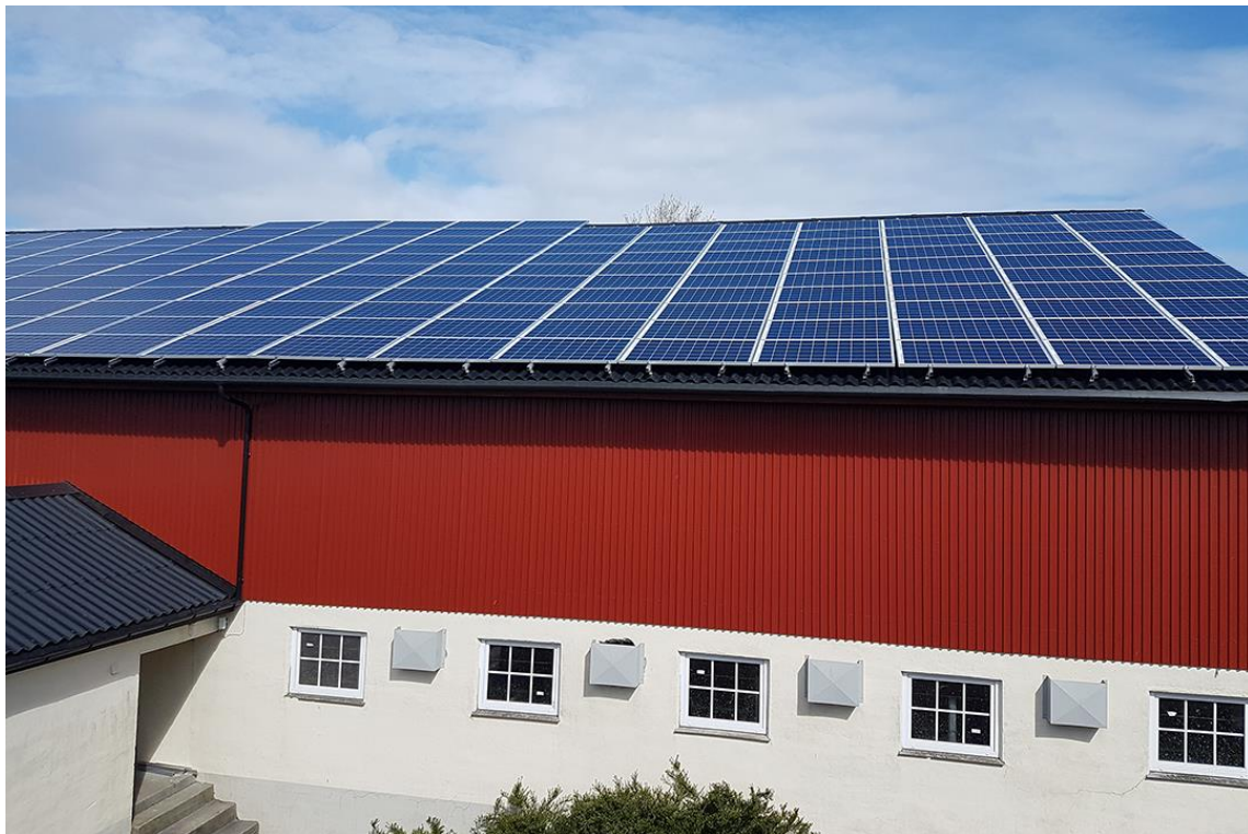
Figure 8: Solar panels on barn roof.
