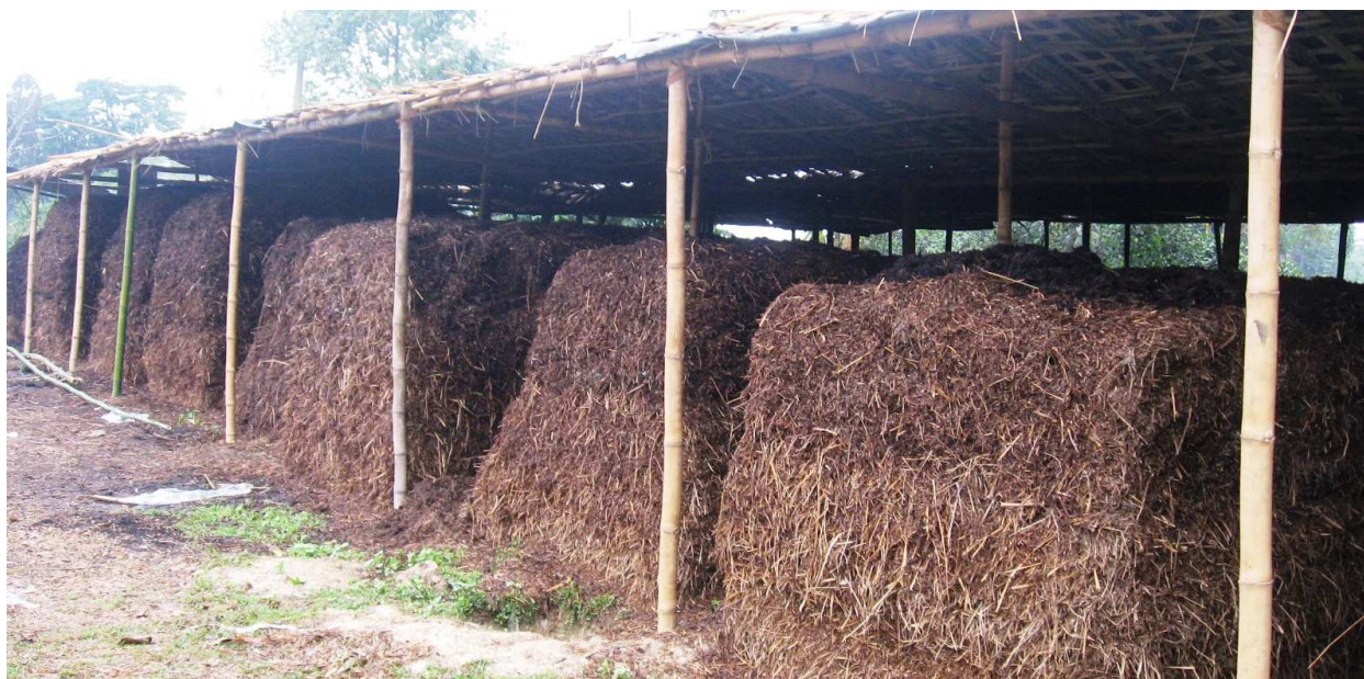
Pic 8: Novcom composting shed at W. Jalinga Tea Estate, Asam, India.
