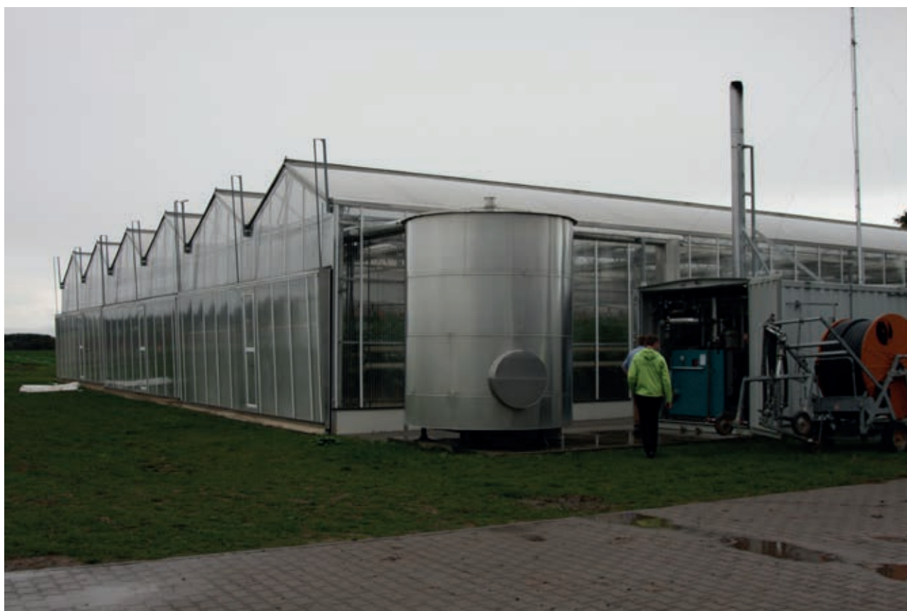
Figure 1.1 A typical greenhouse/glasshouse structure, in this case with a renewable heating boiler.
