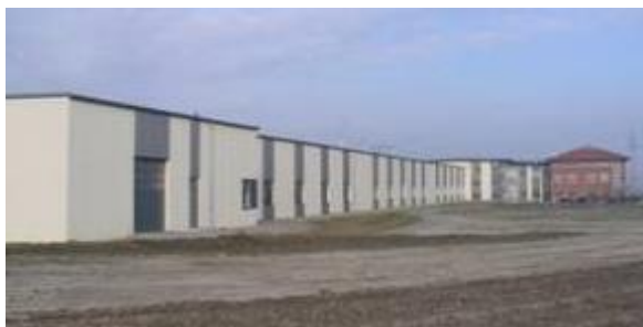
Figure 6: New construction of production plant and office building in 2004
