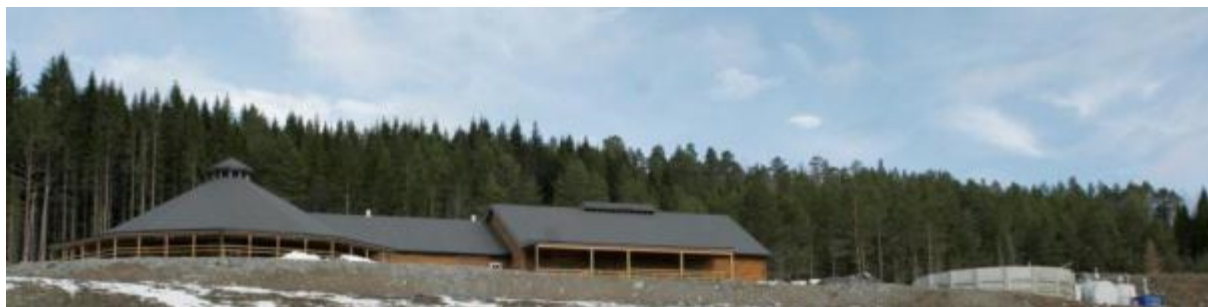
Figure 2.1. The new building for the dairy herd at Tingvoll Farm (to the left), with manure storage in an open concrete tank (right). To the right of this tank, the biogas digesters may be seen. Later, a house was built over the digesters. Photo by Anita Land, November 2010.
