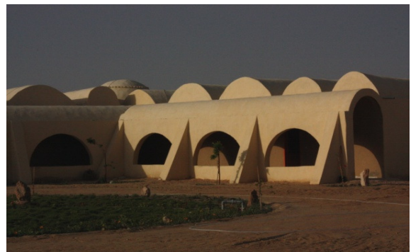
Figure 22. The Sinai farm buildings.
