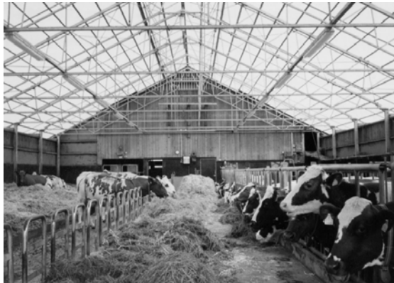
Figure 1. Some cold loose housing barns have a greenhouse structure and the roof is made of see-through acrylic plates.
