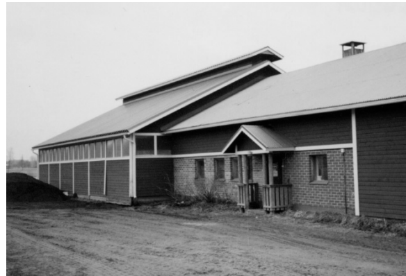
Figure 2. It is relatively common to build the CLHB joined to the old stanchion barn where the milking takes place.
